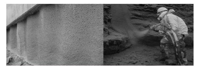
Types of finishing to sprayed concrete -
